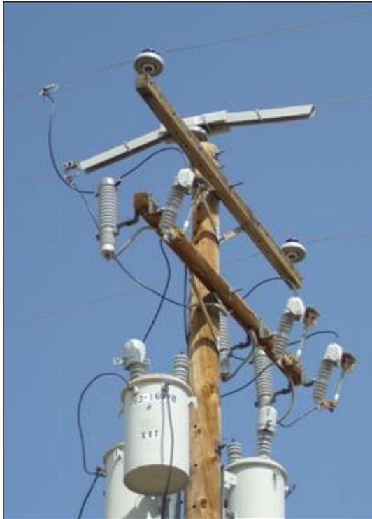
Retrofitted pole with equipment (transformers, cutouts, arresters) and insulator cover
